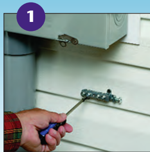
1 Attach grounding bridge to substrate. (Mounting screws not provided.)
