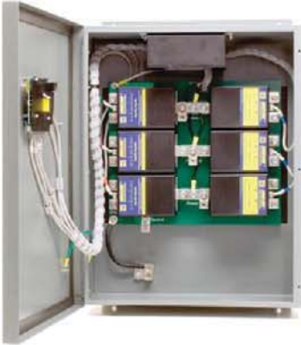
External Modular L-L Enhanced SPD with Sine Wave Tracking Module
